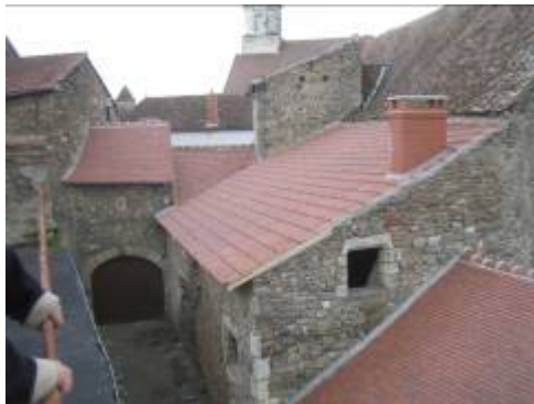
Nos 3 & 5. La Maison de Reine Acquired 2005. Under renovation.
